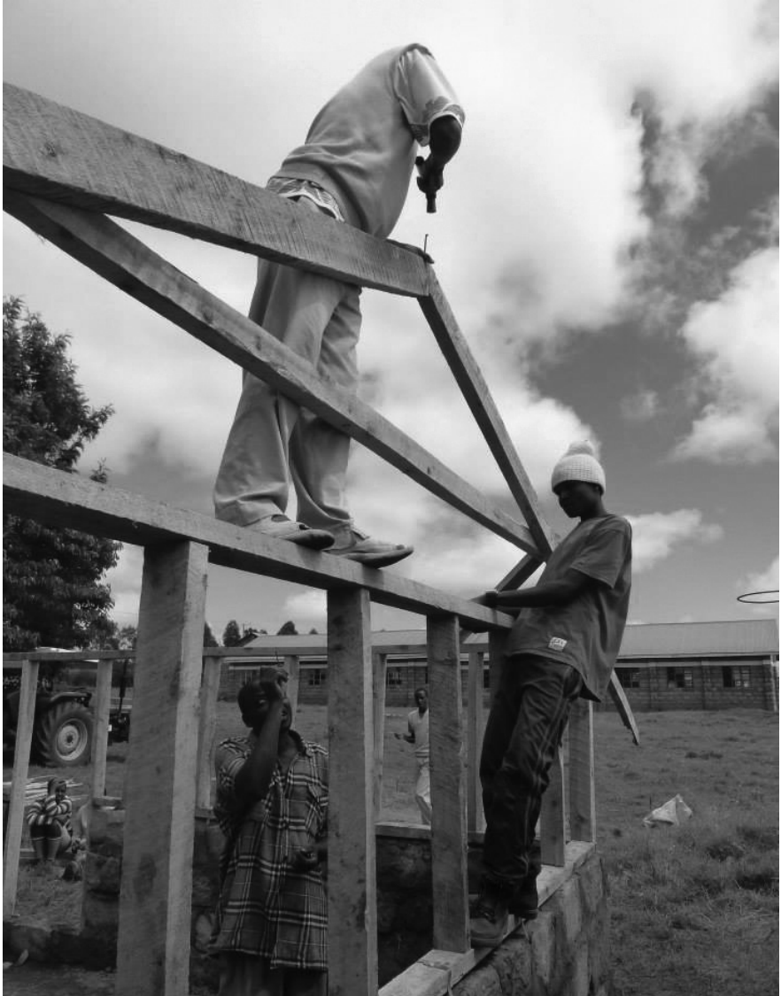
Students Building Chicken House - Legacy Project
